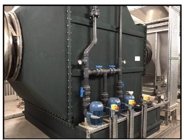
Figure 5 - Vertical Pumps installed on a fume scrubber application
